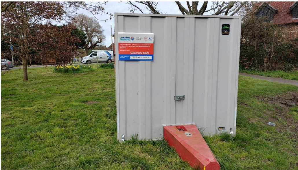
Avonline shed still on grass verge with mud area to left where their vehicle drive over it
